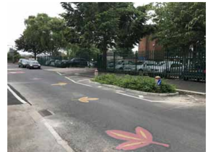
Existing SuDS pod on Embleton Road
